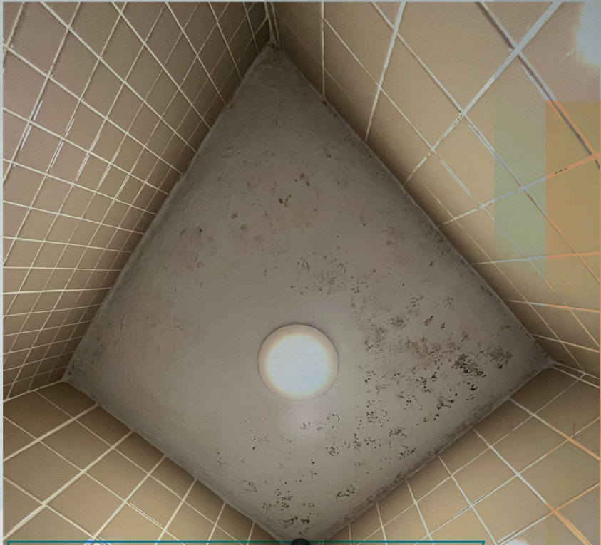
black mold infestation in bathroom (margot j)
