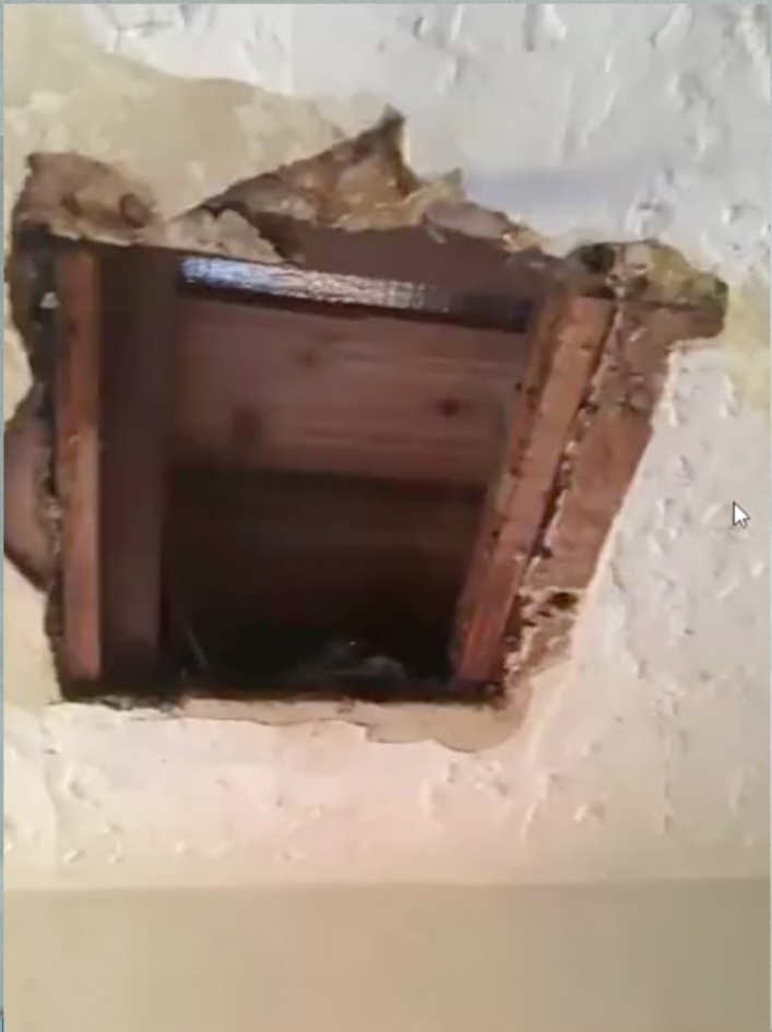
interior hole, living room ceiling (theo k)
